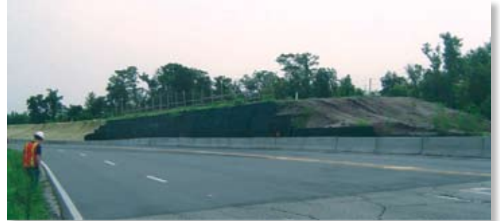
Figure 5. Surcharge to strengthen weak soil remaining after grout injection
