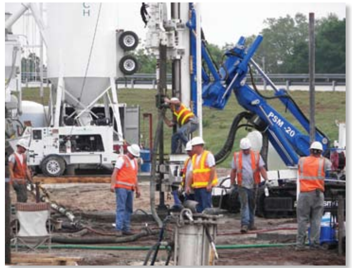
Figure 4. Sinkhole grouting operation at the I-4 and Maitland Boulevard Interchange
